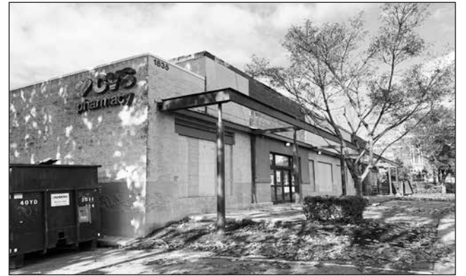
CONSTRUCTION CONTINUES ON NEW CVS PHARMACY
