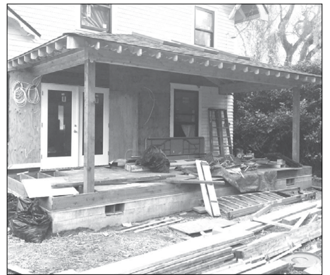
A NEW BACK PORCH IS UNDER CONSTRUCTION.
