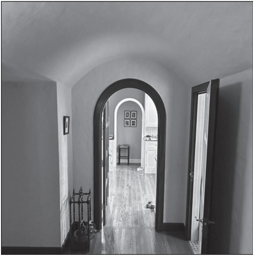
PLASTERED WALLS IN THE HALLWAY, WINDOWED ROOM, AND STAIRWAY CONTAIN MASTER CRAFTSMAN FRED SHEARER'S HAND-DONE COVES AND CORNICE WORK.
