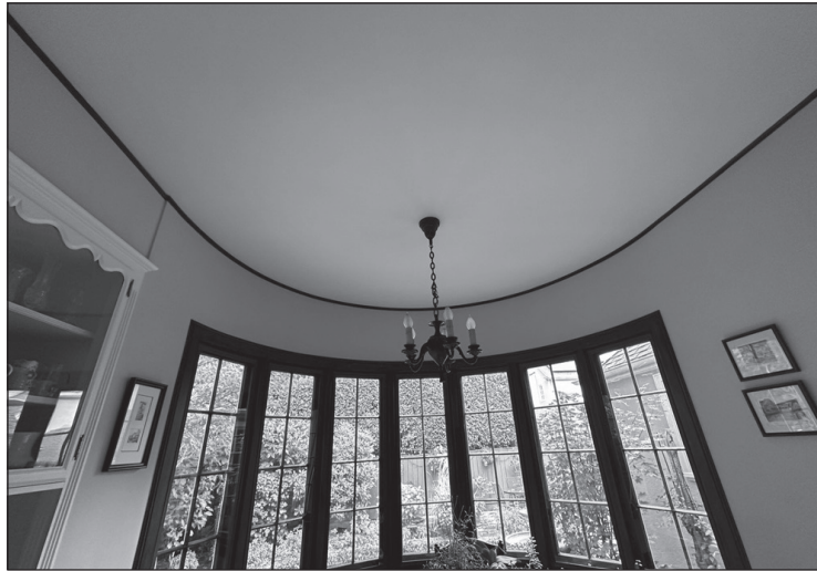
PLASTERED WALLS IN THE HALLWAY, WINDOWED ROOM, AND STAIRWAY CONTAIN MASTER CRAFTSMAN FRED SHEARER'S HAND-DONE COVES AND CORNICE WORK.
