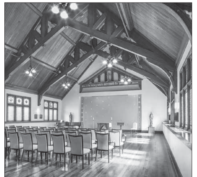
AN ACCENT WALL THAT HAD BEEN PAINTED OVER WAS RESTORED, AND WOOD TRIM AND STAINED GLASS WINDOWS WERE REFURBISHED.
