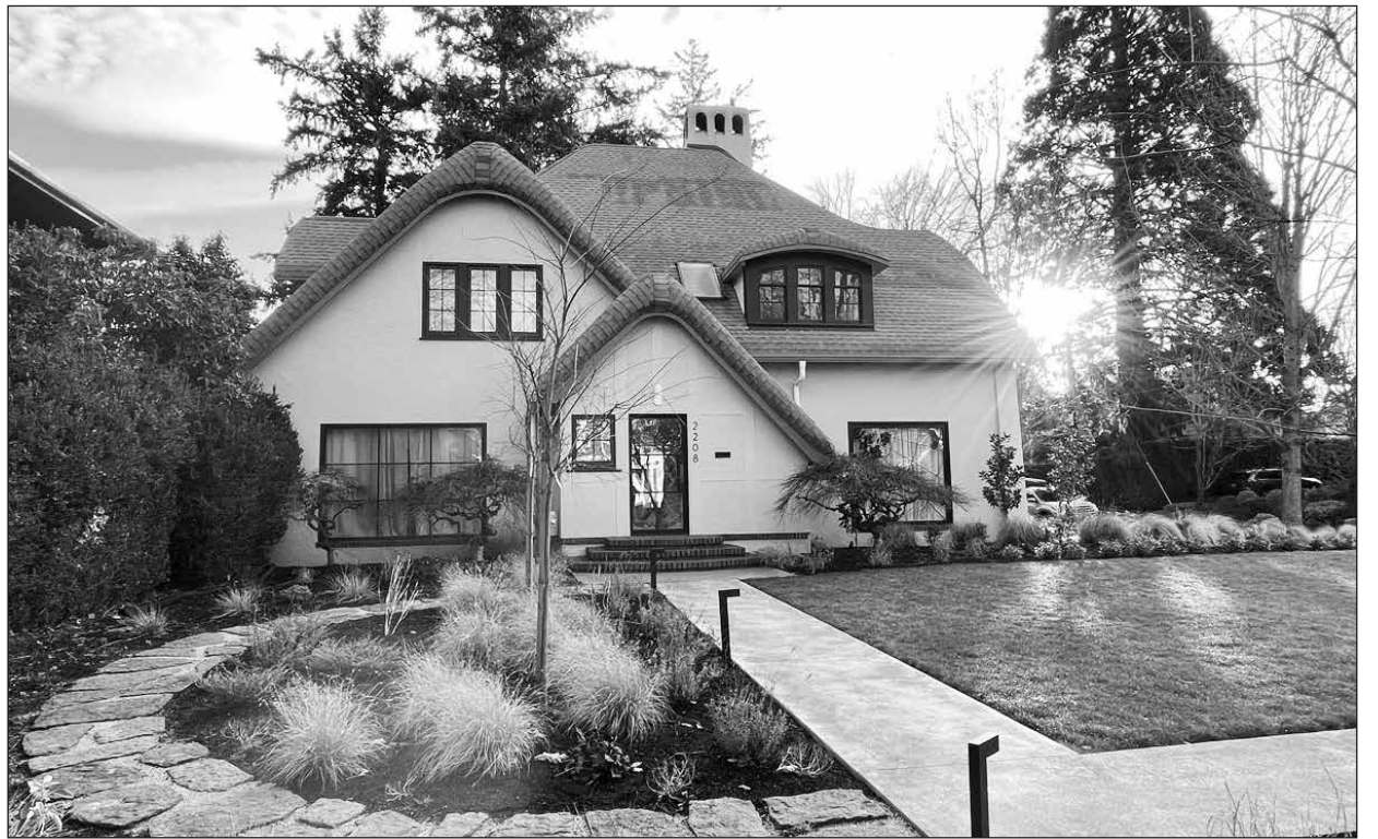
THE FARRINGTON HOUSE AS IT LOOKS TODAY. LARGE PICTURE WINDOWS HAVE REPLACED THE ORIGINAL MULTI-PANE, FULL-LENGTH WINDOWS, AND TRELLISES ON THE SOUTH AND WEST SIDES HAVE BEEN REMOVED.
