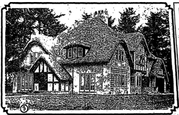
THIS AUGUST 2, 1925 PHOTO RAN IN THE OREGON JOURNAL ILLUSTRATING THE NEARLY COMPLETED FARRINGTON RESIDENCE AT NE 28TH AVENUE AND U.S. GRANT PLACE.
