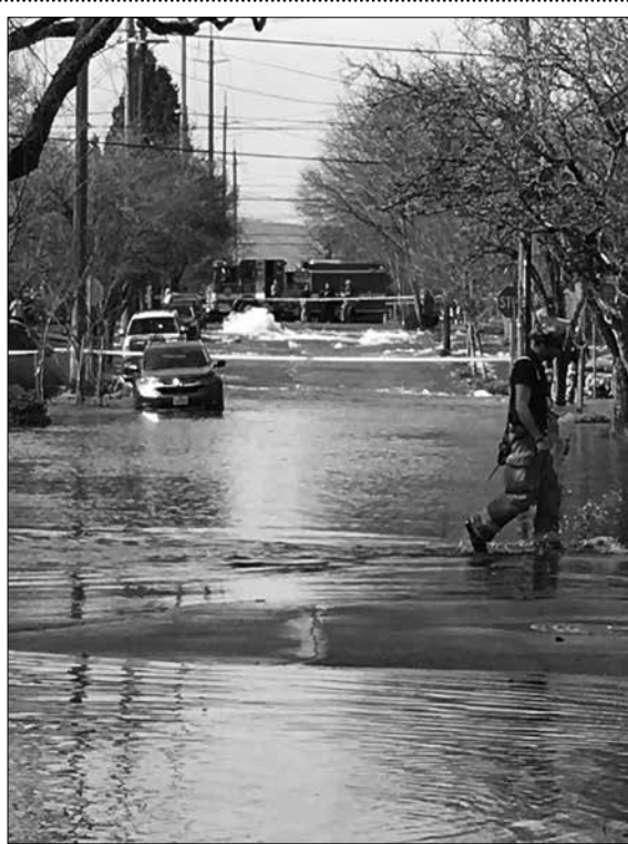
ONE YEAR AGO THIS MONTH: ON SATURDAY, MARCH 16, 2019 A 30-INCH WATER MAIN RUPTURED AT NE 23RD AVE. AND SKIDMORE, FLOODING STREETS AND CAUSING DAMAGE TO NEARBY HOMES AND BUSINESSES.
