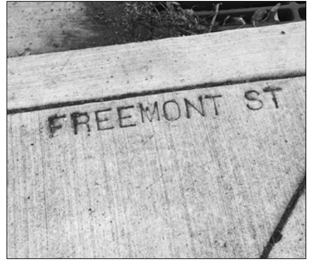
WHEN NEW CURB RAMP WERE INSTALLED ALONG NE FREMONT, THE STREET NAMES WERE RE-ENGRAVED AS WELL. AT NE 28TH, WORKERS ACCIDENTLY PUT AN EXTRA E IN FREMONT - AN IRONIC TOUCH CONSIDERING THE MISPELLING IS DIRECTLY ACROSS FROM A SCHOOL
